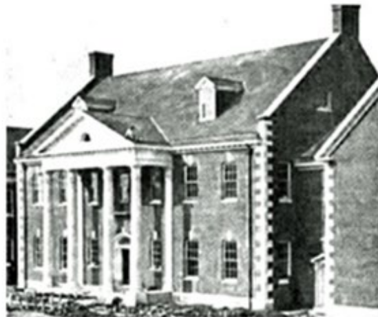
The front of the Kentucky Building during construction in the 1930s.
