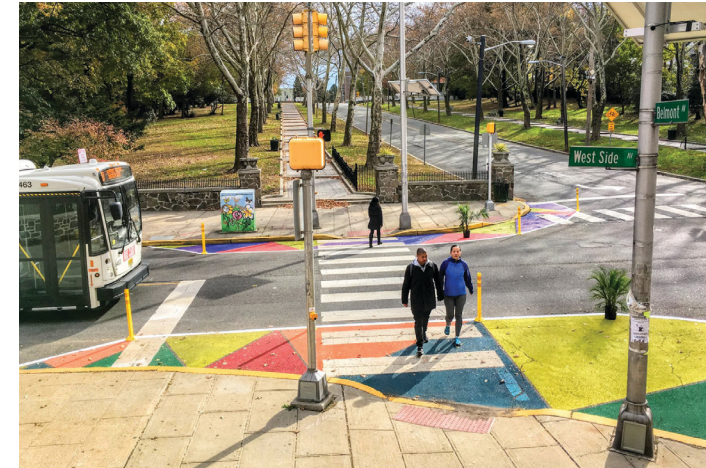
Above: Photo of how simple bollards and paint can transform a crosswalk
